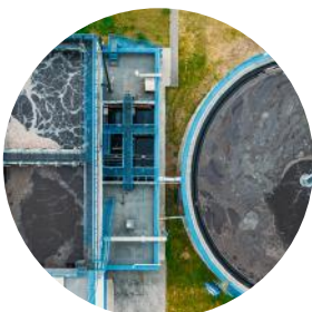
Industrial Wastewater Treatment
