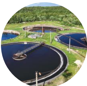
Municipal Wastewater Treatment
